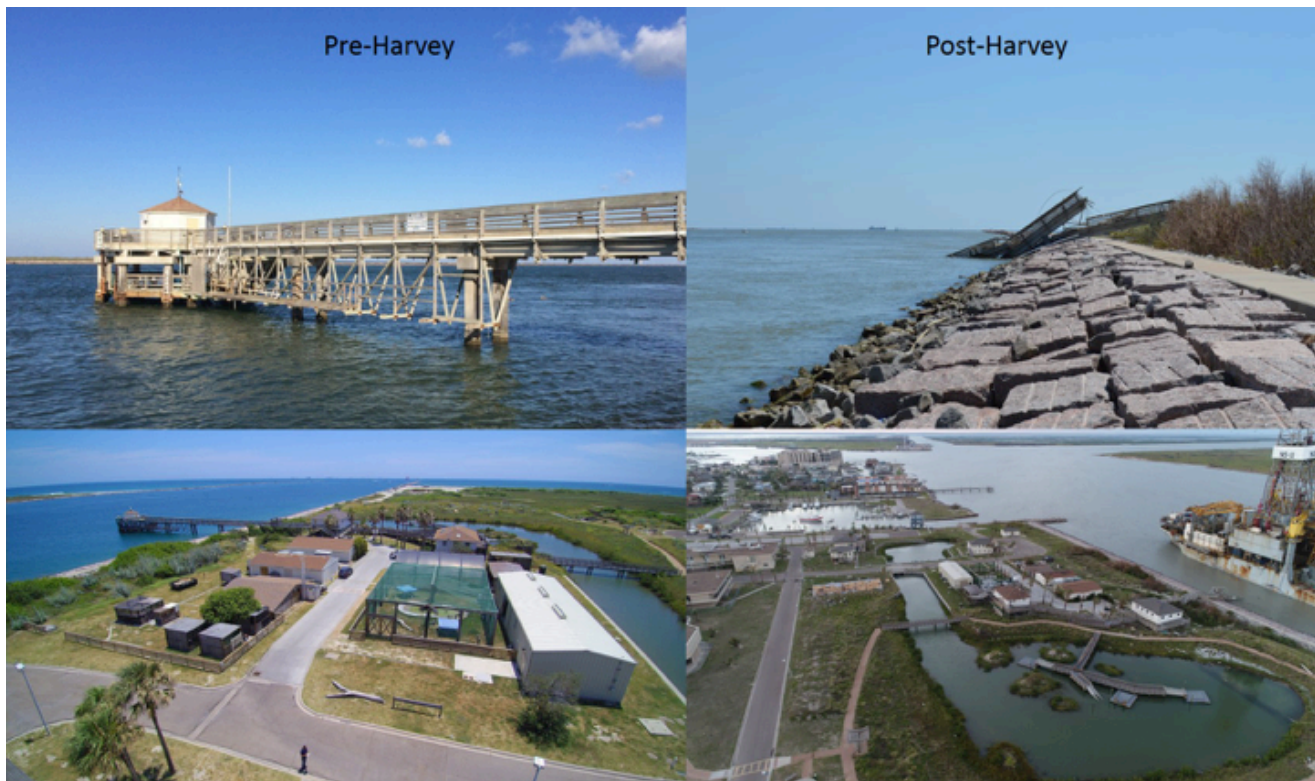
The Marine Science Institute research pier survived the storm, but was crushed by a drilling rig vessel that came lose in the hurricane.
